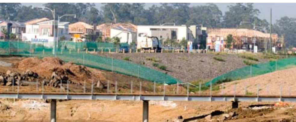
Housing development in western Sydney.
